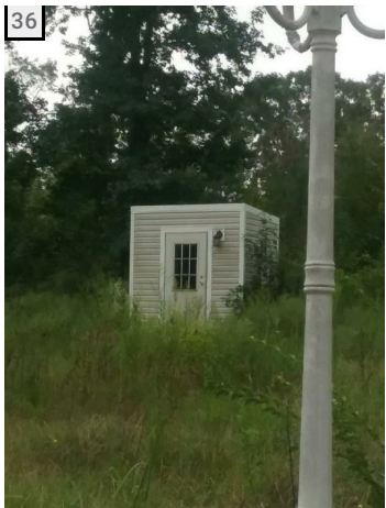
No power supply and filter cartridge is missing
